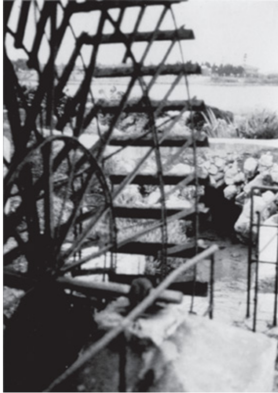
Figure 1.10. Waterwheel on Cephalonia Island built over a sluiceway to generate electricity from inflowing water. The water level drops about 2 meters below sea level by the time it reaches the waterwheel and thereafter drops several more meters before entering a fissure. (Photo by the author)
